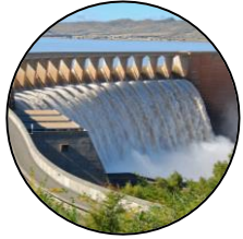
Hydro Power Plants
